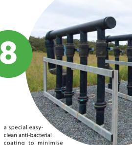
clean anti-bacterial coating to minimise contamination and assist with cleaning and maintenance.
